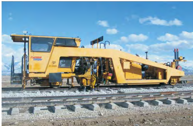
Rail Being Surfaced
