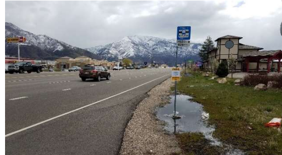
FIGURE 1 - NON-COMPLIANT UTA BUS STOP
